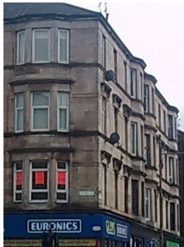
Tenement flats Alison St/Victoria Road
